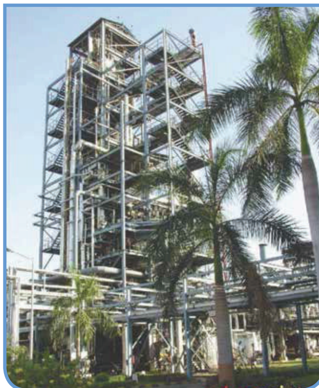
A view of the Company's Phthalic Plant at Ankleshwar, Gujarat
